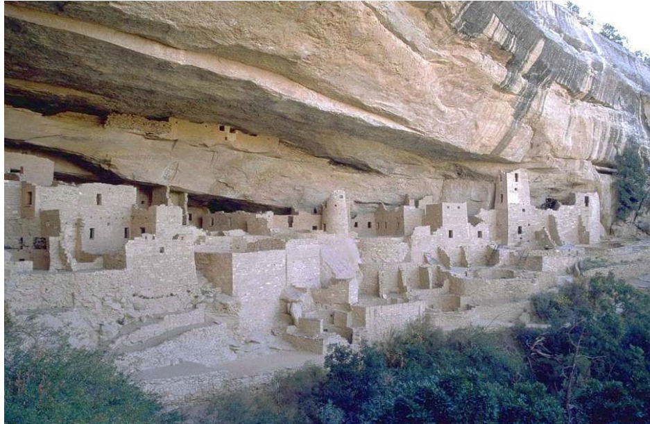
Photograph 2: Mesa Verde, an adobe community built on a superbly located site protected from summer sun, but able to capture solar heat in winter, it was abandoned around 1200, likely because climate change brought on by unsustainable agricultural practises.
