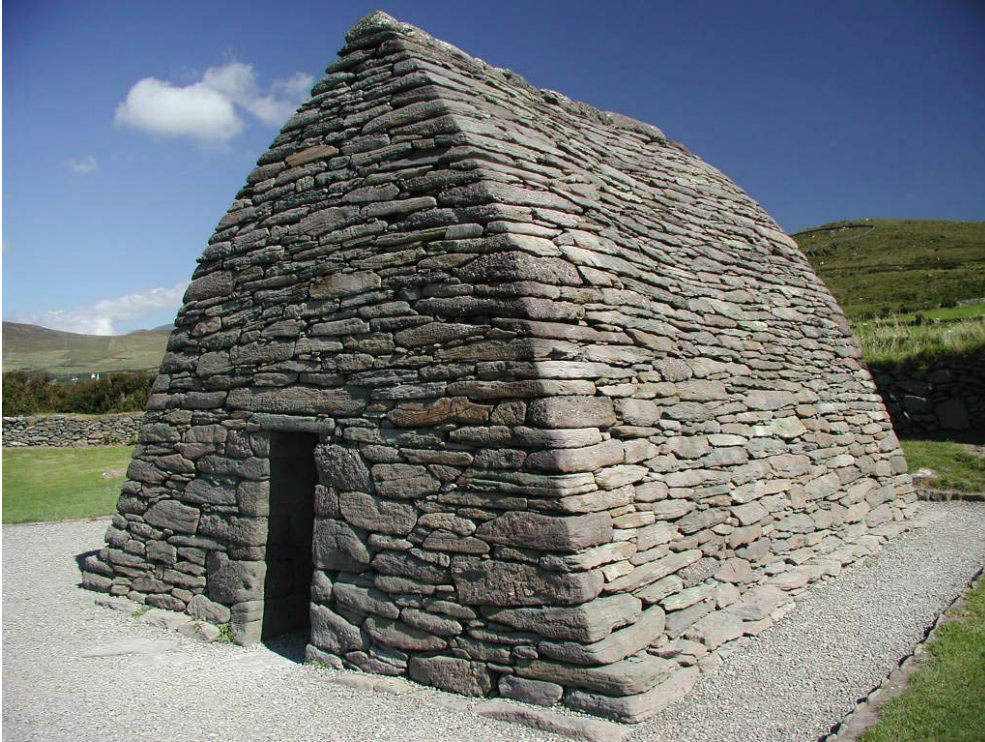
Photograph 1: An Irish Church from 1000 AD composed of just dry-stacked rock. Simple and durable, but hardly comfortable
