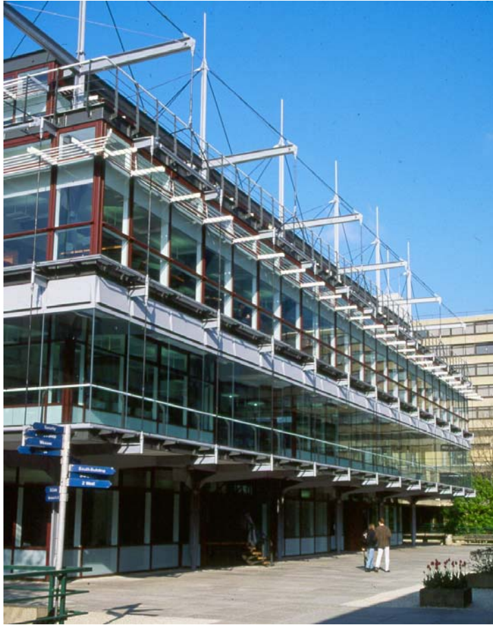
Photograph 5: A recent "high-tech" building enclosure. Poor thermal performance, little solar control, and many sealed joints, this type of enclosure is a serious energy liability and a step backward in indoor climate control.
