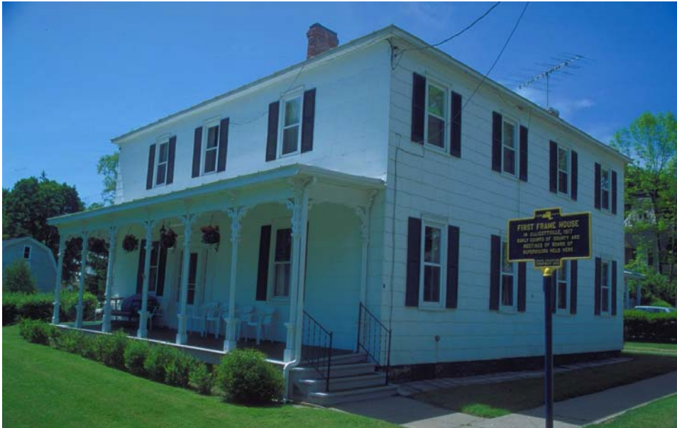
Photograph 4: The first frame building in Ellicottville, NY (1817) is celebrated with a plaque. Such buildings were built with balloon framing, non-standard wood elements and irregular spacings, fastened with both wood pegs and hand forged iron nails.
