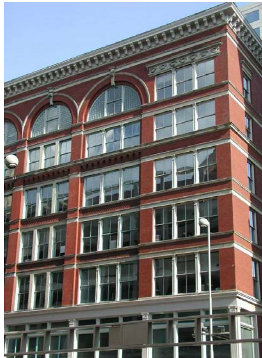
Photograph 3: Solid masonry office with generous window area, and fine detailing. Durable, strong, and functional, with moderate R-value, this type of building was common after the Industrial Revolution
